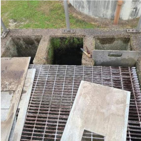
Splitter Box (Slide Gates 1 and 3, removed)
