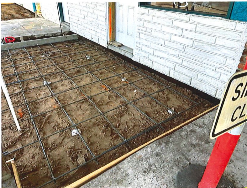
This picture is from a sidewalk that was not tied into the building. The new side walk goes to the edge of the building and has an expansion joint between building and sidewalk so the two are NOT tied in together.'
